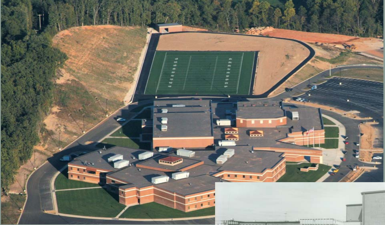
Pictured above is the new 260,000 square foot Camdenton High School, completed in 2007.
